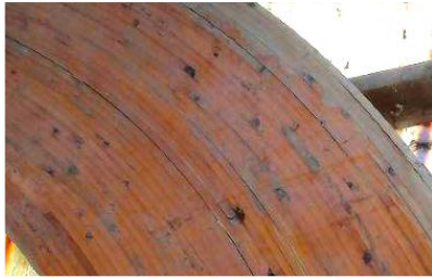
Assessment of cracks
